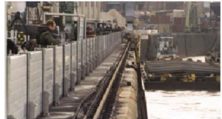
Mobile flood wall Bayer AG, Leverkusen
